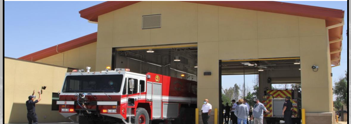
Satellite Fire Station, March ARB, CA
